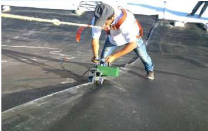
Placement of Geomembrane
