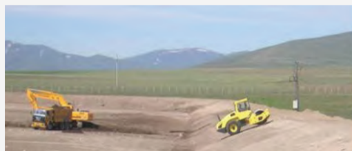
Shape & Compact the landfill basin
