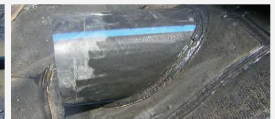
Leachate outflow pipe carefully welded into foil
