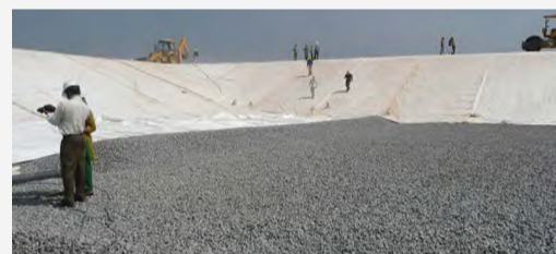
Protective membrane & 50 cm gravel layer
